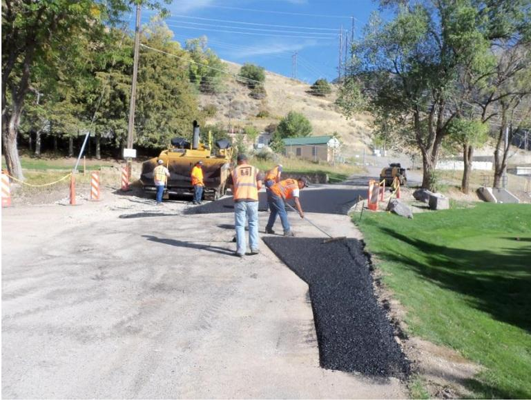
This week on the Valley Segment, crews continued landscaping work and clean up work throughout the segment. LeGrand Johnson Construction, the paving subcontractor, was on site this week repaving all of the roads and sections of pavement disturbed in the valley segment during construction. This included the access road inside the Logan Golf and Country club that leads to the Logan City water tanks.
