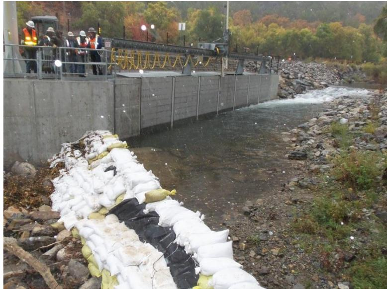
**Flow Test with sand bagged sill wall**
