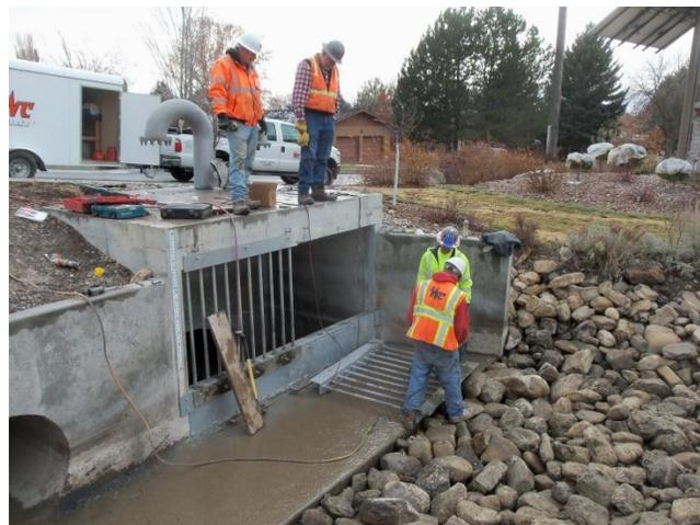
Replacing the original grate on top of the removable steel section
