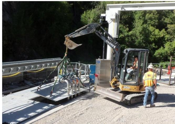
**Pulling out a metal roofing strip in preparation of the neoprene seat installation**
