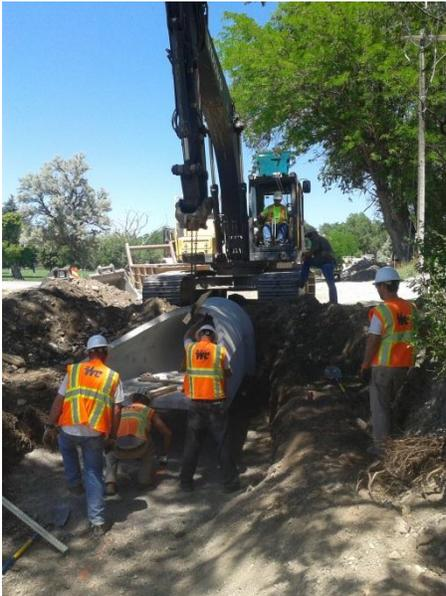
**Installation of concrete end section**
