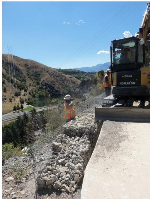
**Construction of the west gabion basket wall**
